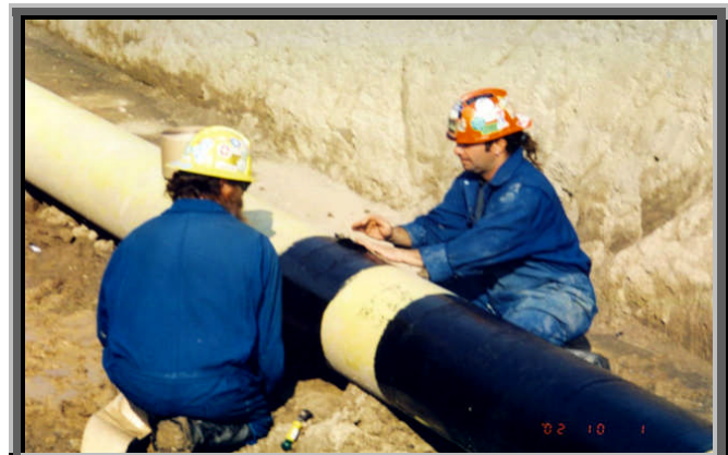
Figure 2-5. Visually Inspect Tape Wrap Installation. Remove Excess Wrinkling and Air Pockets. Recoat.
