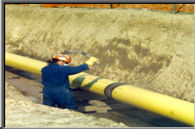
Figure 2-1. Remove Old Coating.
