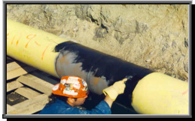
Figure 2-3. Apply Liquid Primer.
