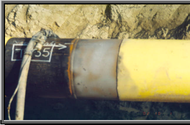
Figure 2-2. Minimum Power Tool Clean.
