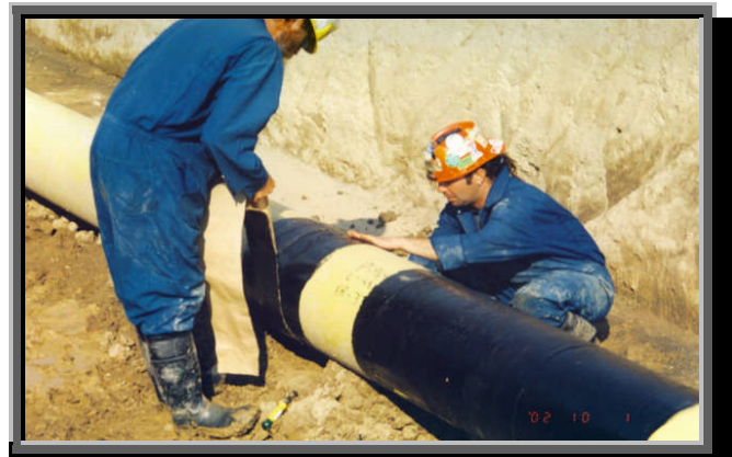
Figure 2-4. Let Primer Dry. Apply KEMA Series 60.
