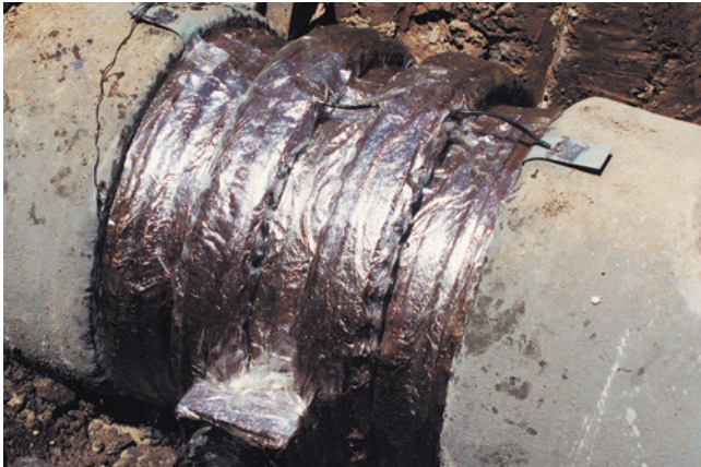
Poly-Ply outerwrap is a multi-layer version of plastic wrap. It helps keep a separation between the tape and the soil.
