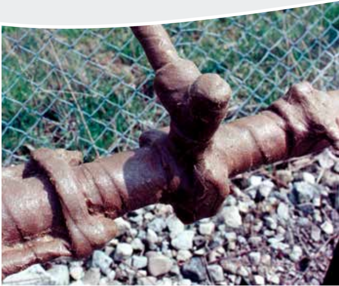
Wax-Tape® #1 anticorrosion wrap applied to coupling, street tee and leak clamp.
