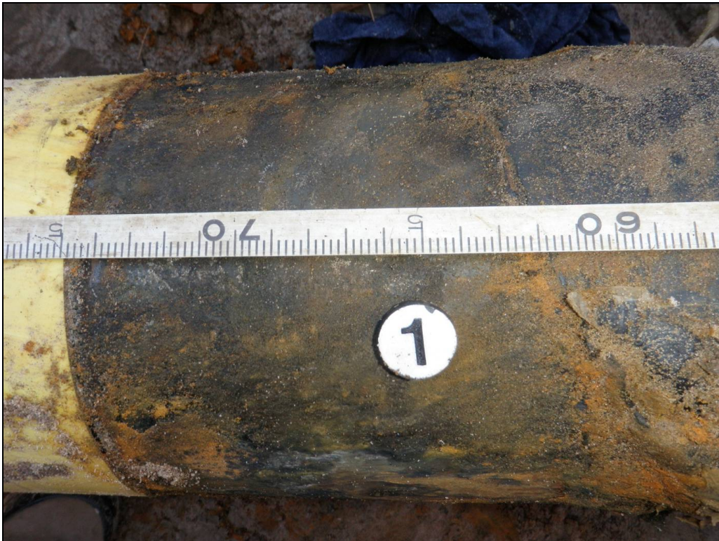
Figure 8: Dig Site #4. Bare Areas at Weld
