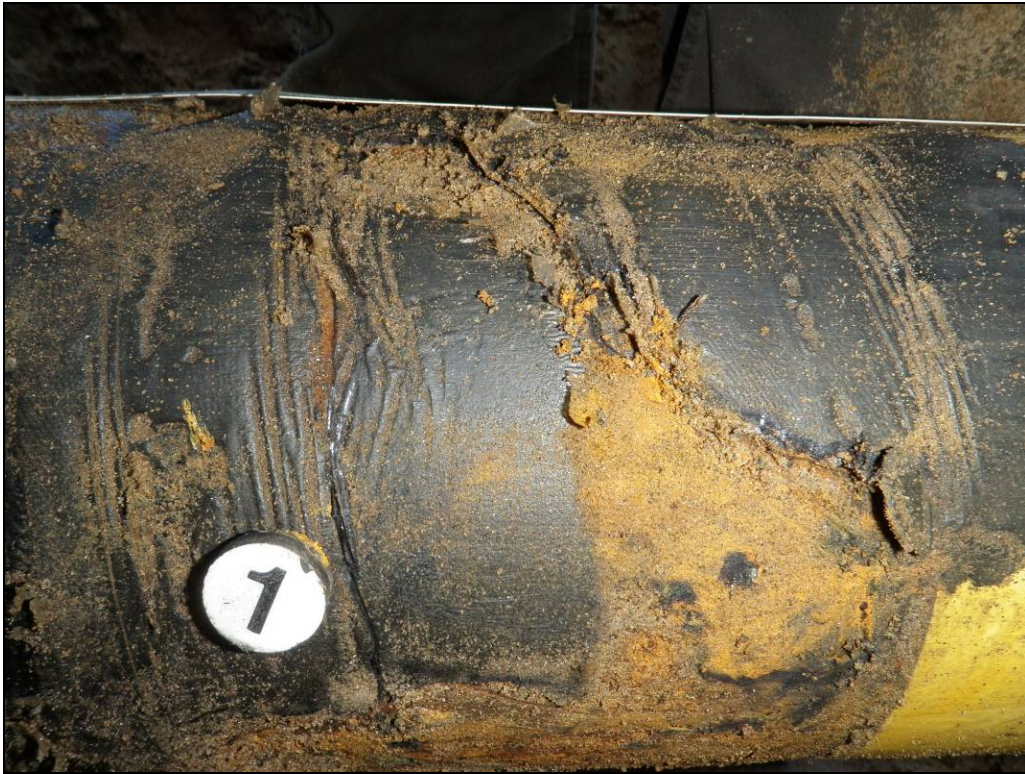
Figure 7: Dig Site #1. Bare Areas at Weld
