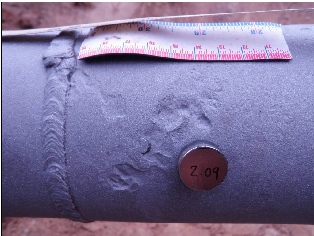
Figure 6: Pitting at Dig Site #6
