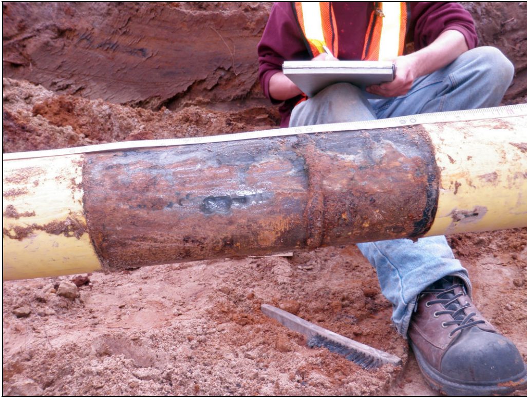
Figure 9: Dig Site #6. Bare Areas at Weld
