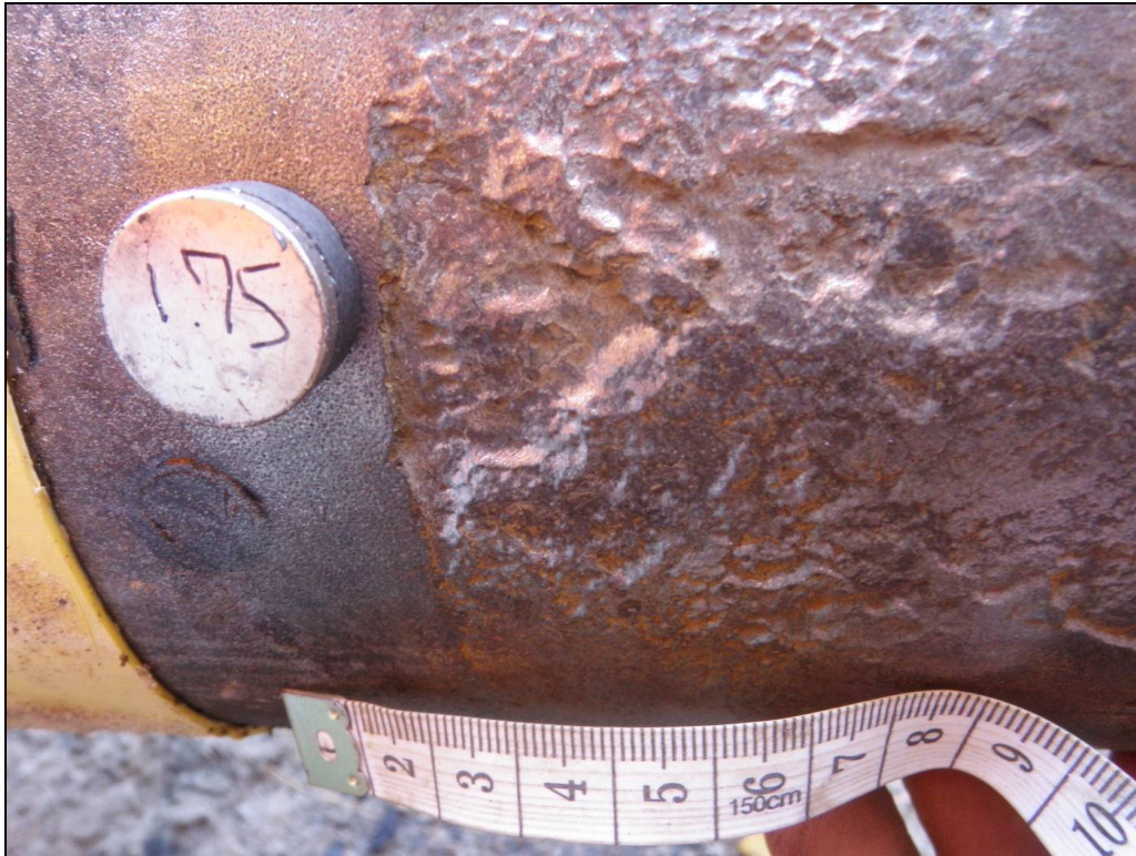
Figure 5: Pitting at Dig Site #4
