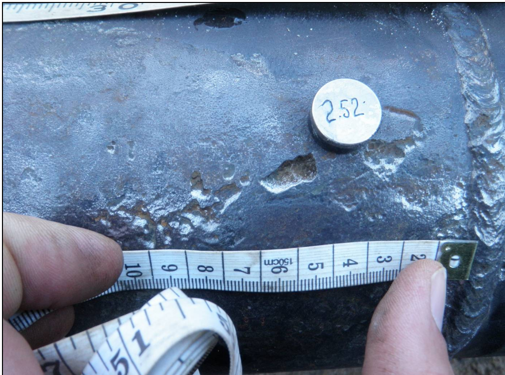
Figure 4: Pitting at Dig Site #1
