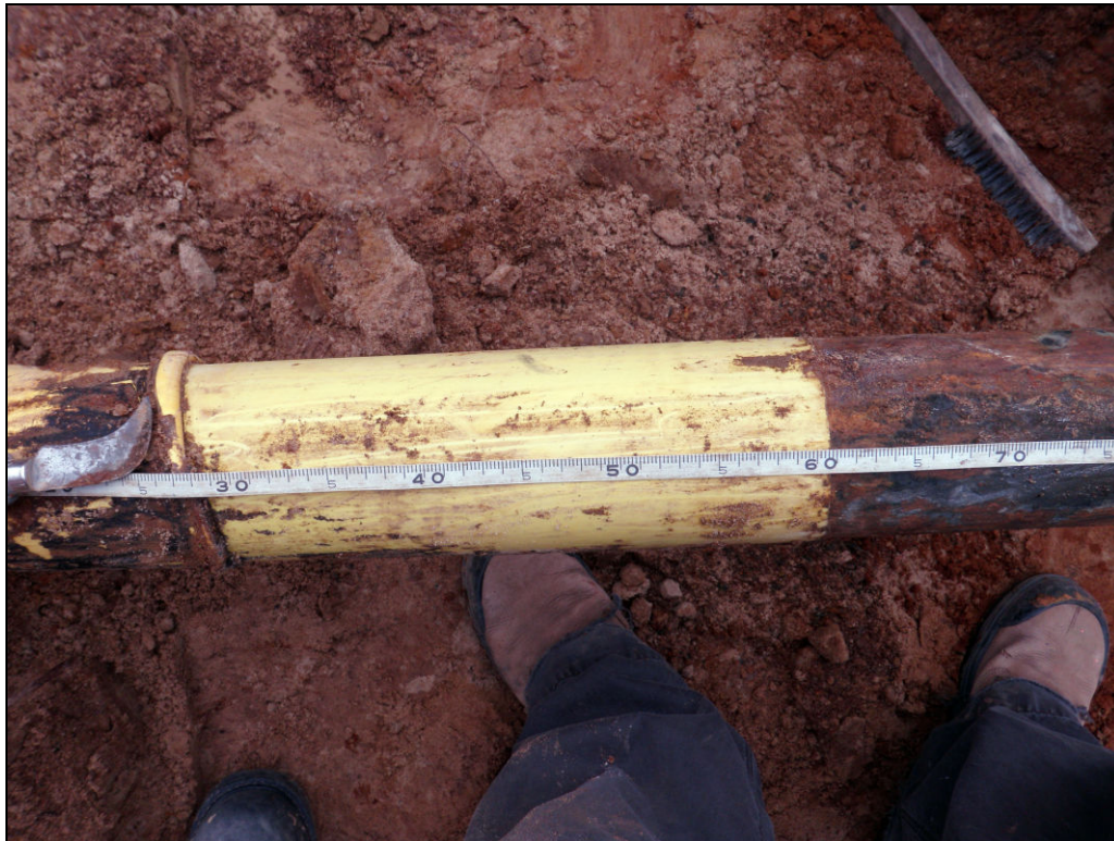
Figure 10: Dig Site #6. Damaged Factory Coating in Vicinity of Weld
