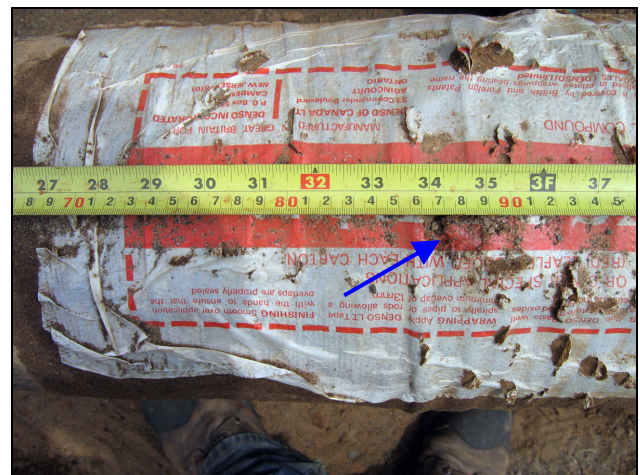
FIGURE 9 • DE #2. Connection of Depleted Magnesium Anode.
