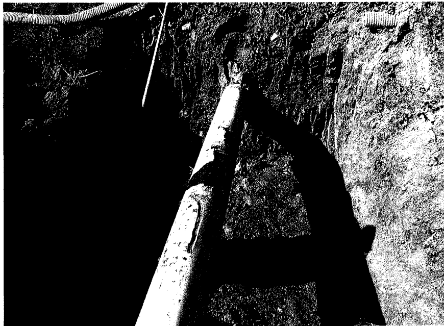
Figure 15. Leamington North Tie Over. Coating Damage at Chainage 181.85m
