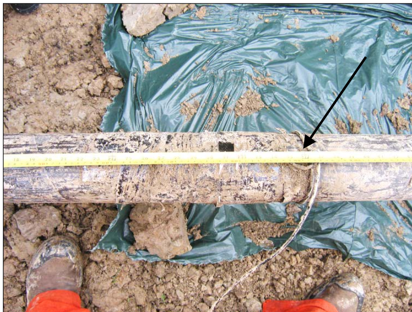
Figure 5: Magnesium Anode Connection
