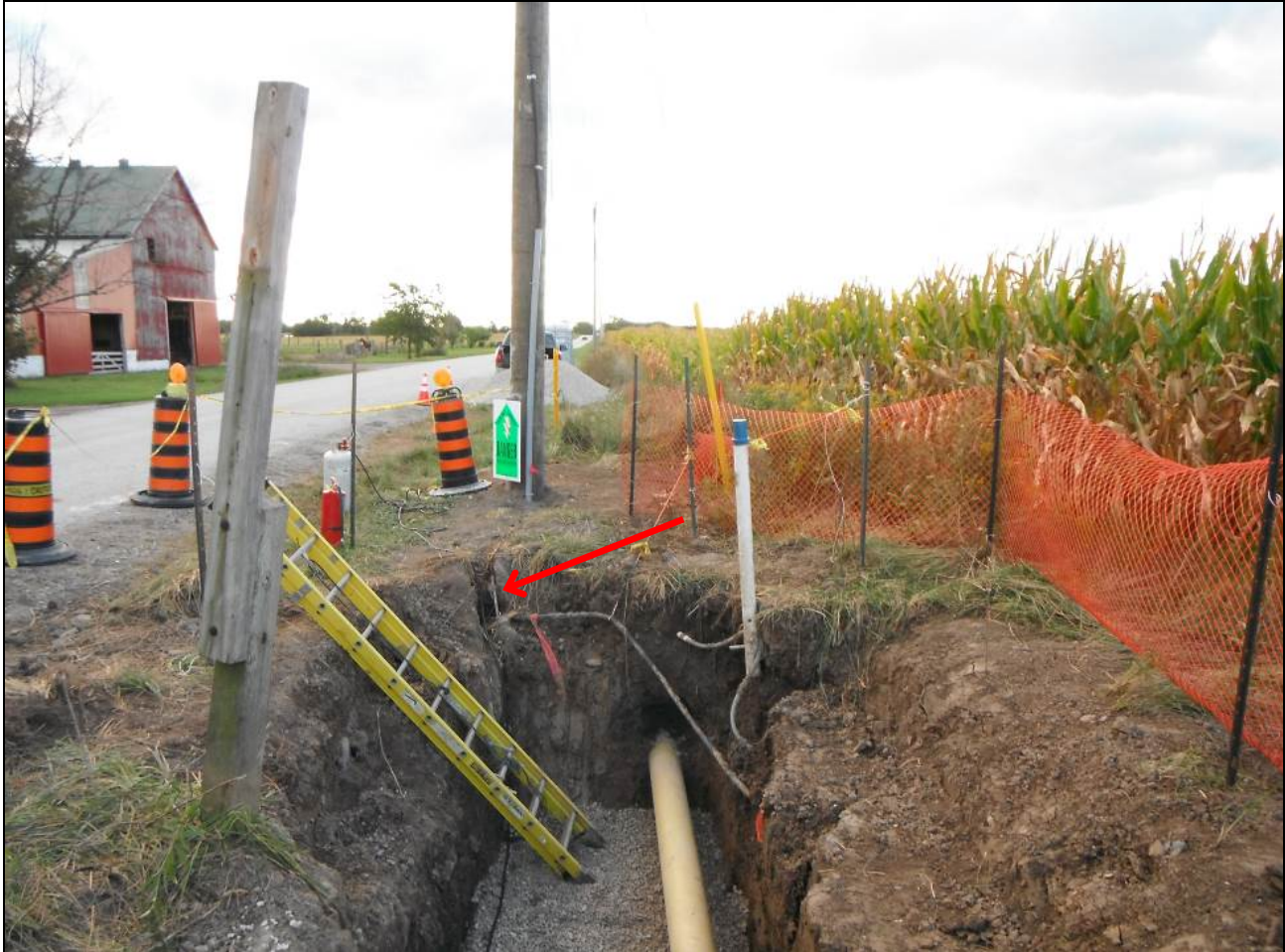
Figure 7: DE#2 Open Trench. Looking South. Buried Grounding Rod
