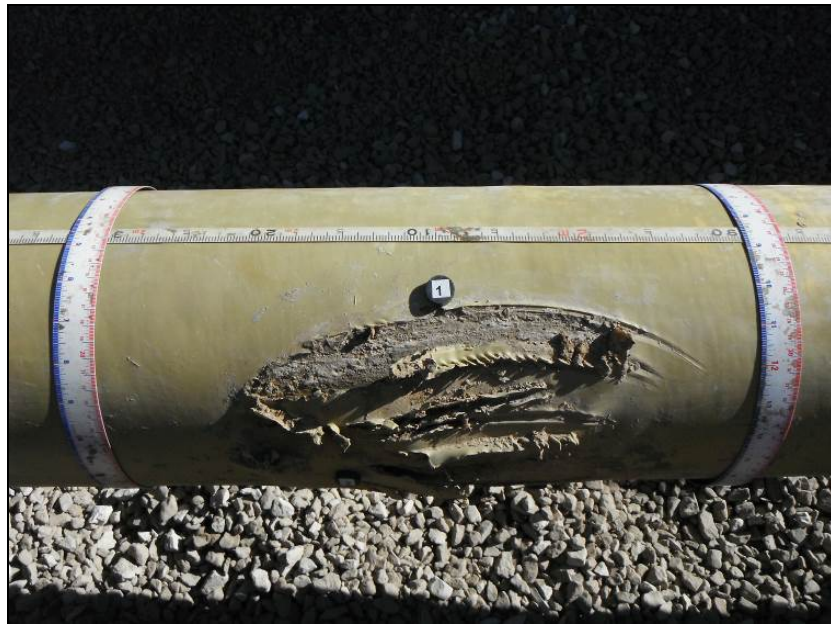
Figure 3: DE#3. Third-Party Coating Damage. Holiday #1
