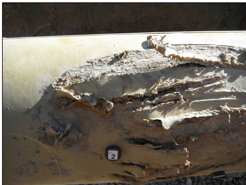
Figure 4: DE#3. Third-Party Coating Damage. Holiday #2
