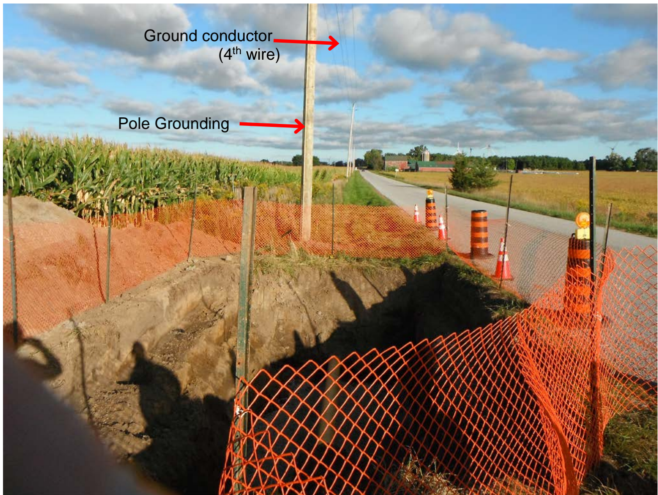
Figure 8: DE#1 Open Trench. Looking North. Powerline Ground Conductor and Pole Grounding
