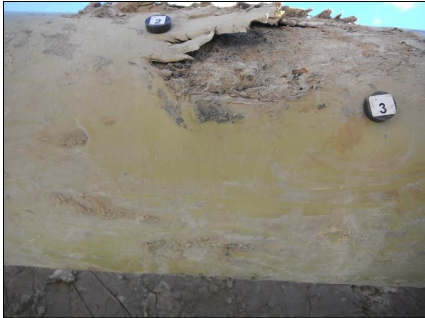
Figure 5: DE#3. Third-Party Coating Damage. Holiday #3
