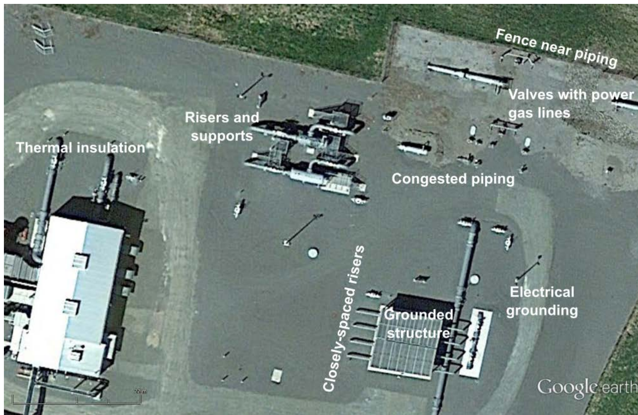
Figure 1: Satellite image showing challenges typical to a compressor station.
