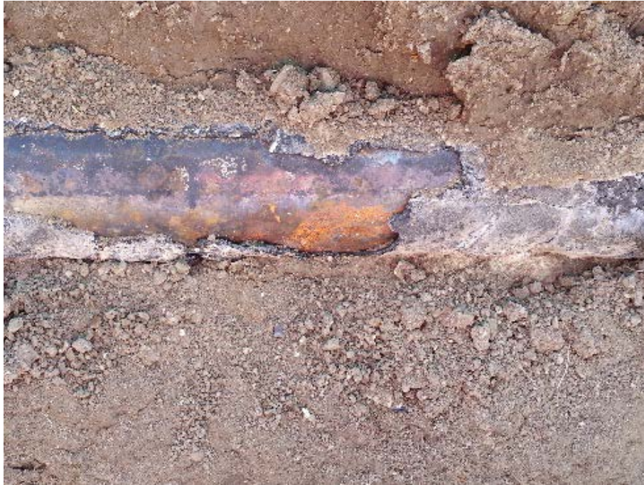
Figure 9: Initial exposure of NPS 4 pipeline, prior to coating collapse.
