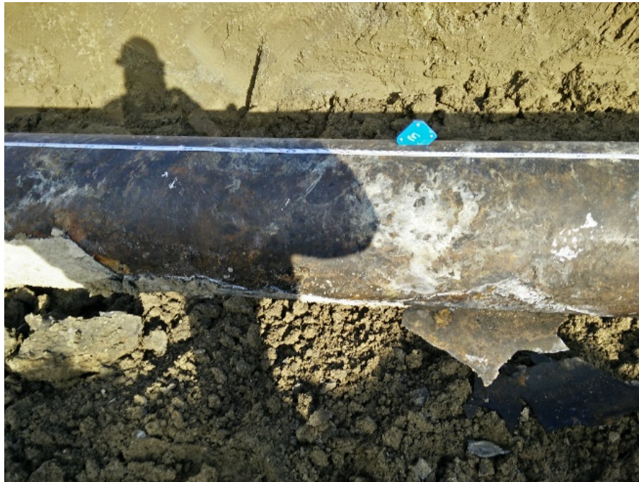
Figure 8: Extremely poor coating and calcareous deposits were observed on the NPS 12 pipeline.
