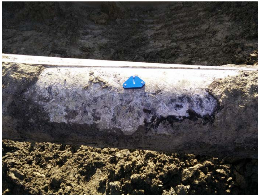
Figure 10: Calcareous deposits on NPS 12 pipeline.
