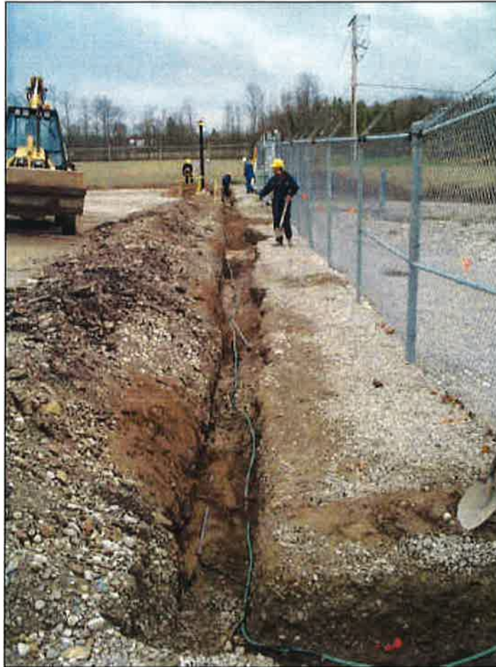
Figure 3 – Installation of Station Perimeter Grounding System
