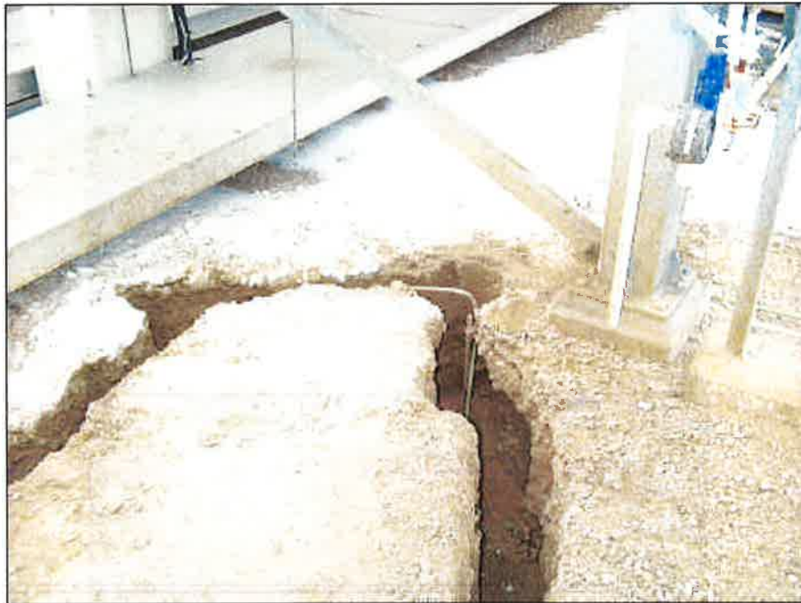
Figure 4 – Removal of Copper Grounding System
