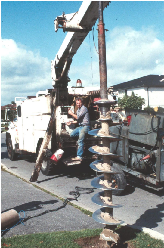
Figure 20 – Augering Hole Above the Watermain
