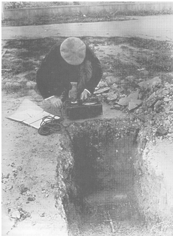
Figure 4 – Early Testing for Stray Current Activity (courtesy of East Bay Municipal Utility District, Oakland, CA)
