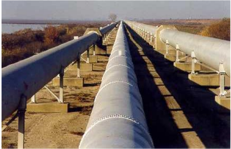
Figure 17 – View of the Mokelumne Aqueducts. Middle pipe is the original aqueduct installed in the early 1920's (photo courtesy of East Bay Municipal Utility District, Oakland, CA)
