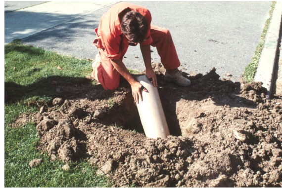
Figure 21 – Lowering Magnesium Anode into the Augered Hole
