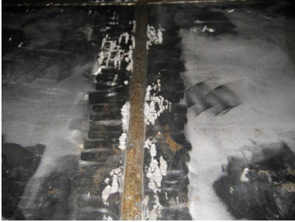
Figure 2: Pitting damage on the side of a vertical weld seam after 18 months operation. Base metal pitting also visible at upper right area of photo.
