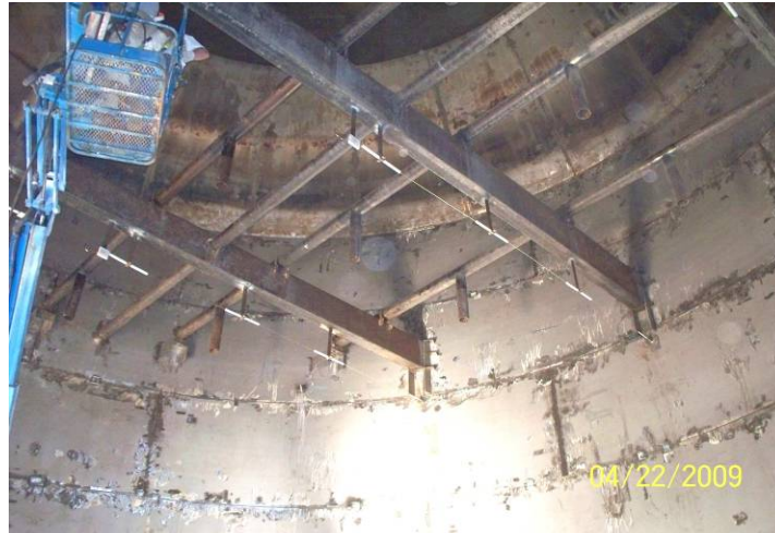
Figure 10: Anodes Installed beneath Air Sparger Support Steel.
