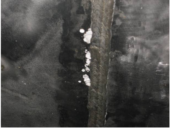
Figure 3: Closer view of pitting corrosion at Heat Affected Zone (HAZ) of weld.
