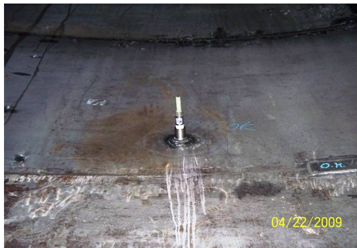
Figure 11: Reference Electrode Installation
