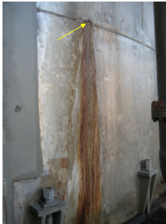
Figure 1: Through-wall corrosion damage after 18 months of putting a new scrubber into operation. Note brown staining below the damage.
