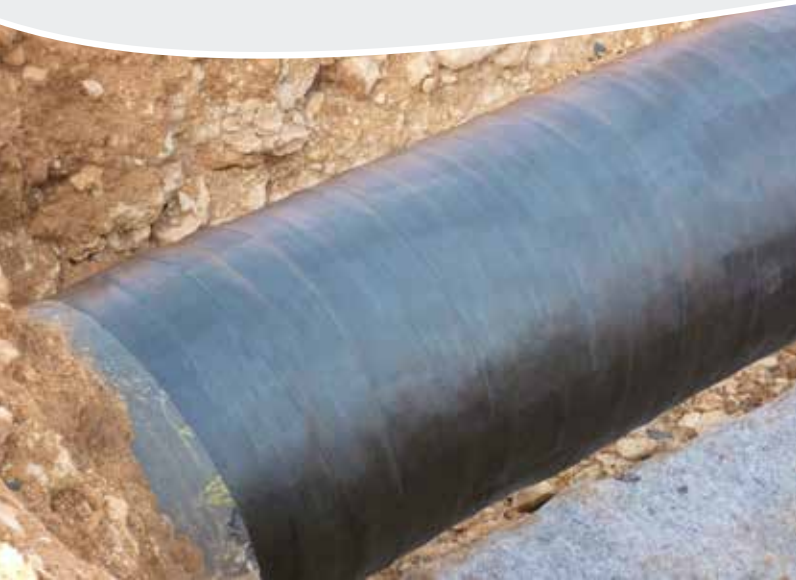
MCO ® 110 outerwrap is specially formulated to quickly provide a hard outer shell. The photo on the right shows MCO 110 outerwrap applied over Trenton's Wax-Tape ® HT-3000 high-temperature anticorrosion wrap. The combined wrap system provides both mechanical and anticorrosion protection.
