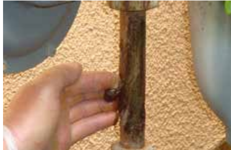
5. Pay special attention to applying primer in and around all angles and threads.
