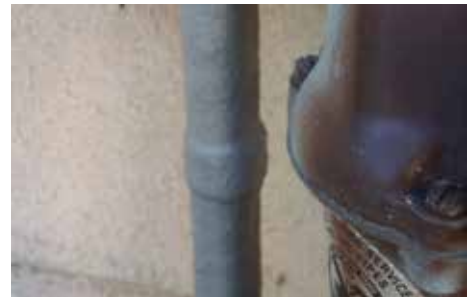
9. Inspect your work. Make sure all desired areas to be coated are completely covered. Remove and re-apply if needed.
