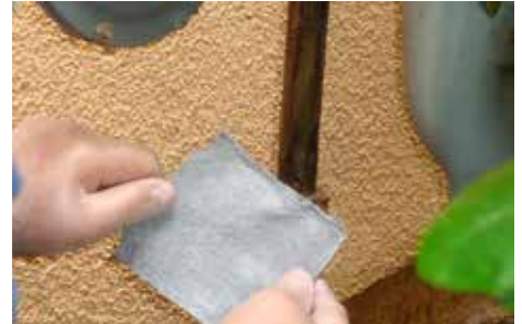
6. Wipe hands clean of primer. Remove pad of Trenton Wax-Tape® wrap from package and remove the backing paper.
