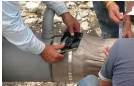
Seal-Wrap banded securely in place and buckles being covered with small squares of Double-Faced Adhesive.
