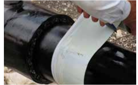
First layer of Double-Faced Adhesive is applied to the carrier.
