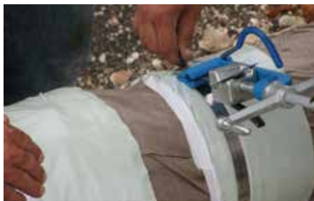
Last wrap of Double-Faced Adhesive with release paper not removed, banding
