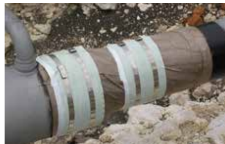
Completed installation showing wrapping secured with two bands.
