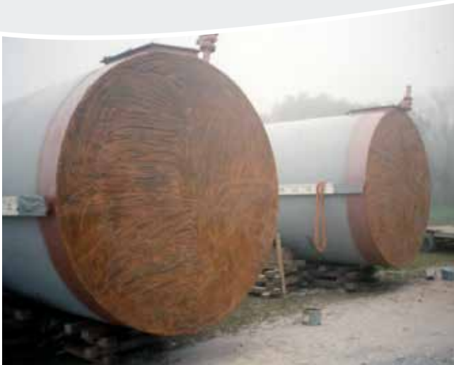
Temcoat 3000 applied to pipe surface. It will then be wrapped with Poly-Ply™, Guard-Wrap® or Wax-Tape®.
