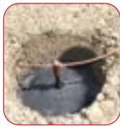
2. Ground enhancement material, GEM or Quickfill
