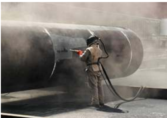
Conventional grit blasting
